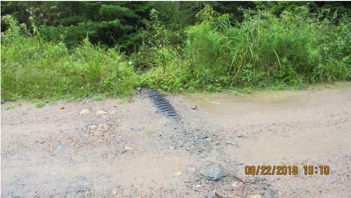
Woodstock Road exposed culvert. (Source: EDM)
