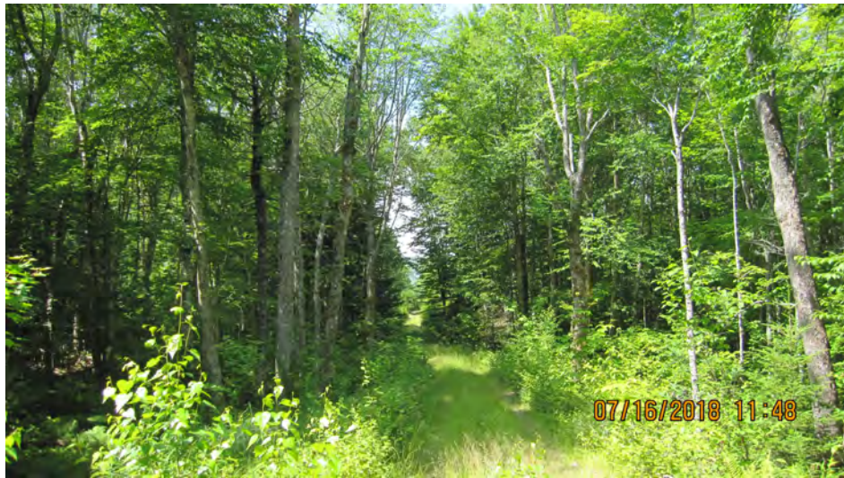
Private park road - lower driveway in need of widening. Large trees to be kept. (Source: EDM).
