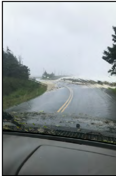
Washout of a road near crescent beach
